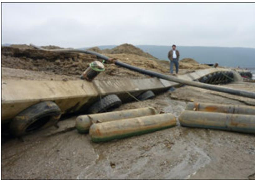
Figure 23: Lateral spreading damage from the 2010 magnitude 8.8 Chile earthquake. (Technical Council on Lifeline Earthquake Engineering - TCLEE)
