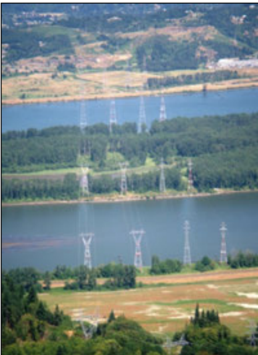
Figure 51: High voltage electrical transmission crossing over the Columbia River just west of Longview, Washington. (DOGAMI photo)
