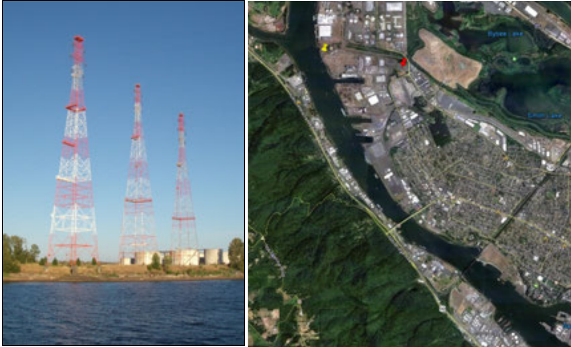
Figure 28: Two towers in the CEI Hub are owned by BPA (center and right in photo on left, yellow pin in NW corner of map on right) and were analyzed in a BPA study conducted in 2008 to have the potential to move 25 feet towards the river during a magnitude 9 Cascadia earthquake. (The tower in the foreground - left-hand side of photo - is owned by an investor-owned utility.) (DOGAMI photo) (map: Google Earth)
