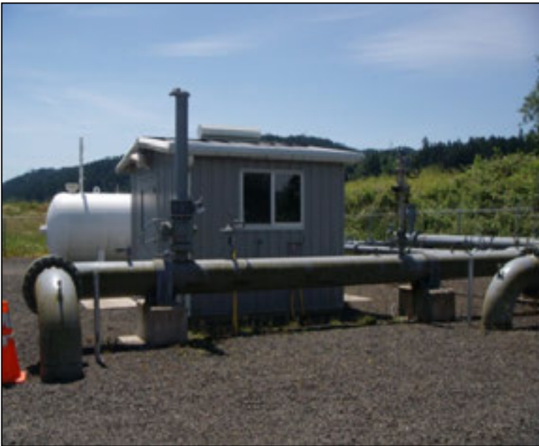
Figure 53: Several liquid fuel and buried natural gas pipelines at the Columbia River and Willamette River crossings just north of the CEI Hub. Photo shows a natural gas gate station on Sauvie Island. (DOGAMI photo)
