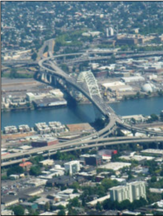
Figure 57: The 1973 Fremont Bridge, part of Interstate 405, crosses the Willamette River and is used for liquid fuel distribution. (DOGAMI photo)
