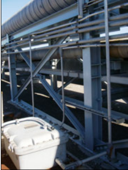
Figure 71: This photo shows an example of an oil company in California that is following best practices learned from other earthquakes. The white box contains an accelerometer that records site-specific data. Having the recorded ground motion data will allow engineers to better understand the performance of the structures at the oil terminal and help them evaluate the structural performance and improve future designs. (DOGAMI photo)
