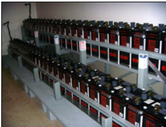
Emergency batteries, as well as other components such as generators and communication devices, should be braced or anchored to withstand Cascadia earthquake. (DOGAMI photo)
