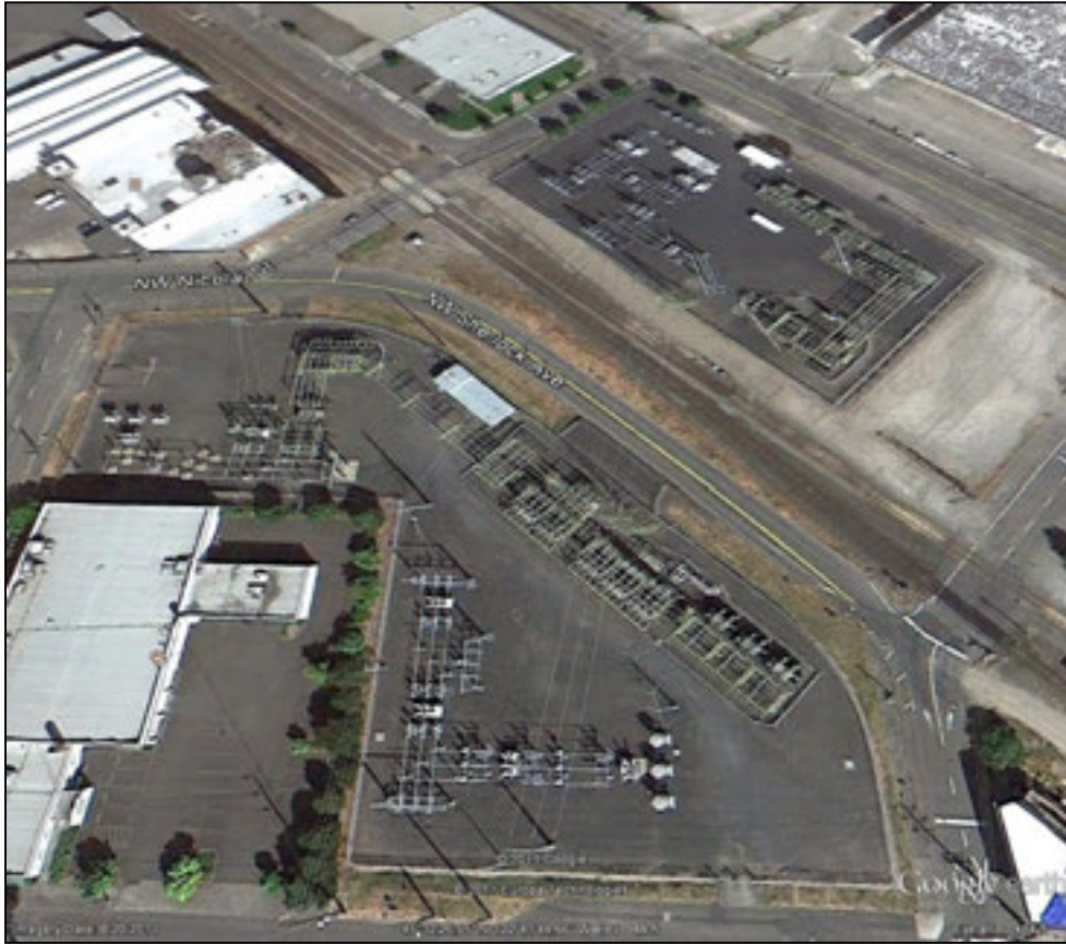
Figure 32: Two large electric substations just south of the CEI Hub on Front Street that are separated by a railroad track (Basemap: Google Earth)
