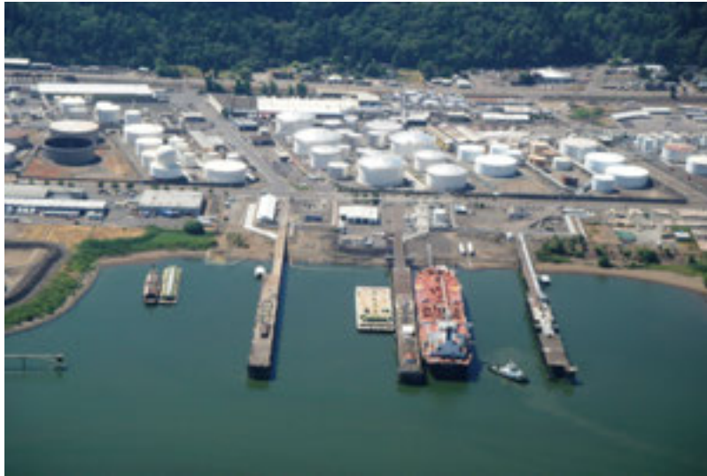
Figure 8: Oil terminals in the southern portion of the CEI Hub. (DOGAMI photo)
